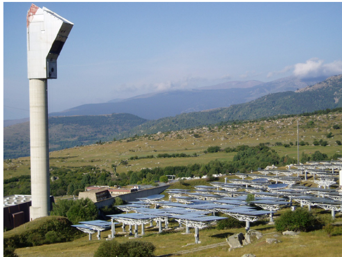
Figure 1: The Thémis CSP tower plant in Targassonne, France. Source: https://commons.wikimedia.org/wiki/File:Themis_2.jpg .
